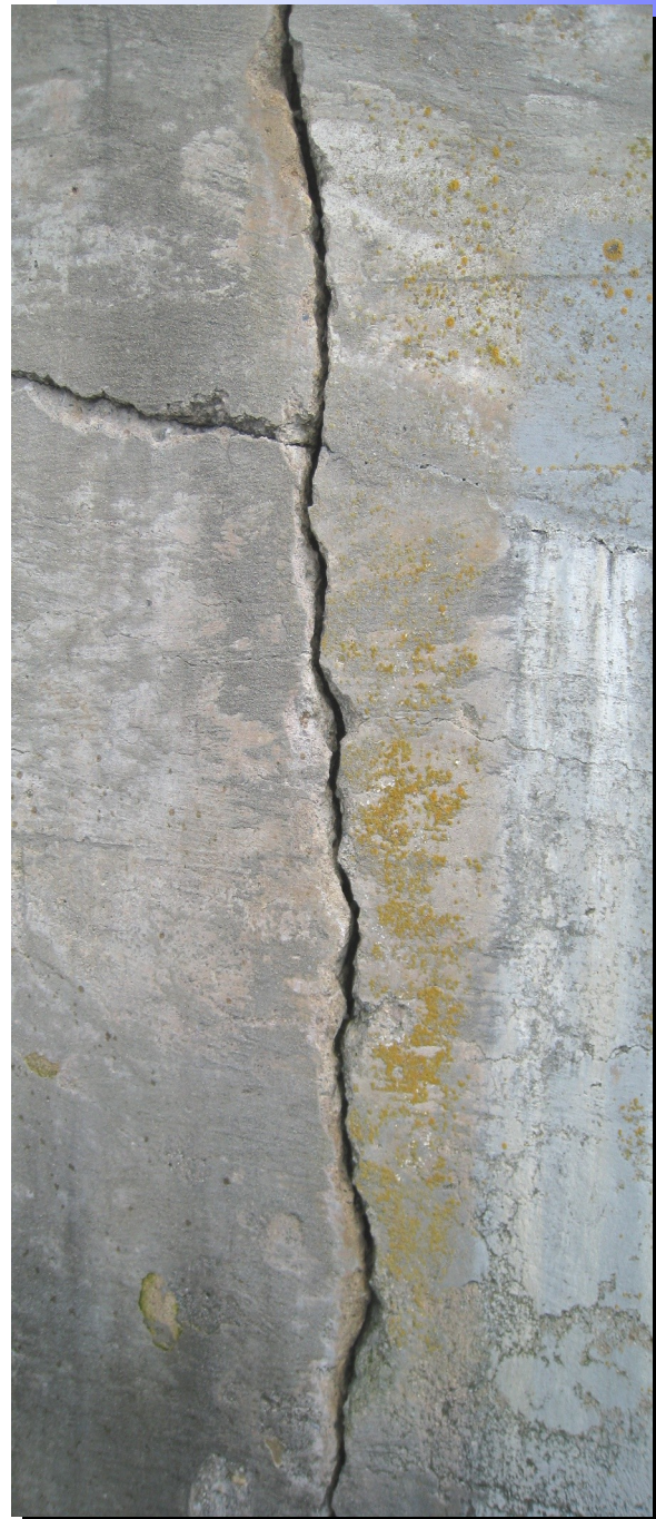
Typical Vertical Foundation Cracking / Zelmer
