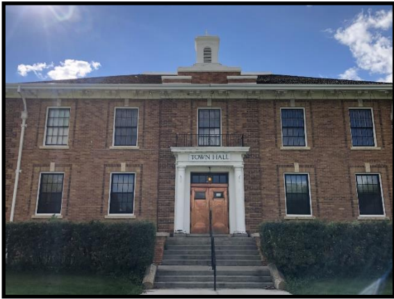
Shaunavon Court House Window Replacement Project – Photo Credit: Town of Shaunavon
